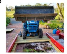
Notice the extreme deflection of the two deck boards under the tires. That is with nothing in the loader. Another reason to use a top mounted deck with the girders directly beneath the tire path. The boards in the picture might actually break if the loader were full of dirt or rocks.
