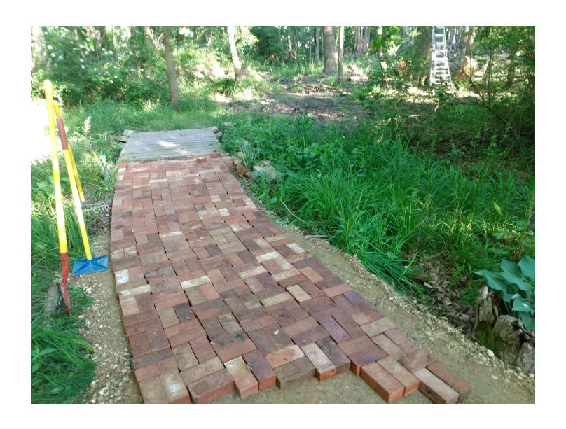
Zoe Ahaghotu Bridge can be seen in the background. At right rear the ladder to the top of the stump of the recently felled large willow oak, site of the future Tree House, can be seen. The bed of compacted RCP can be seen extending beyond the brick pavers.
